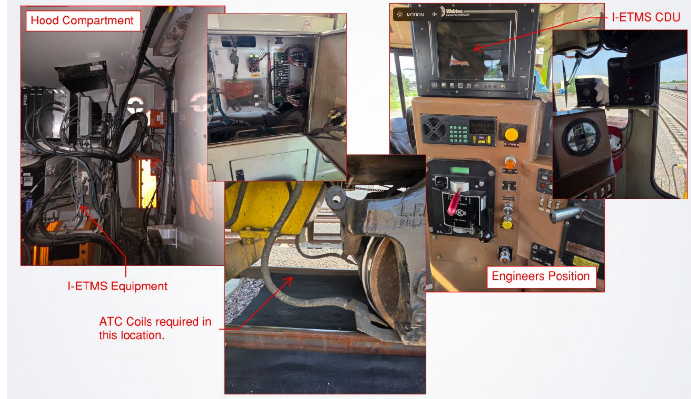
DGNO locomotive survey — existing I-ETMS equipment and required ATC coil location.
