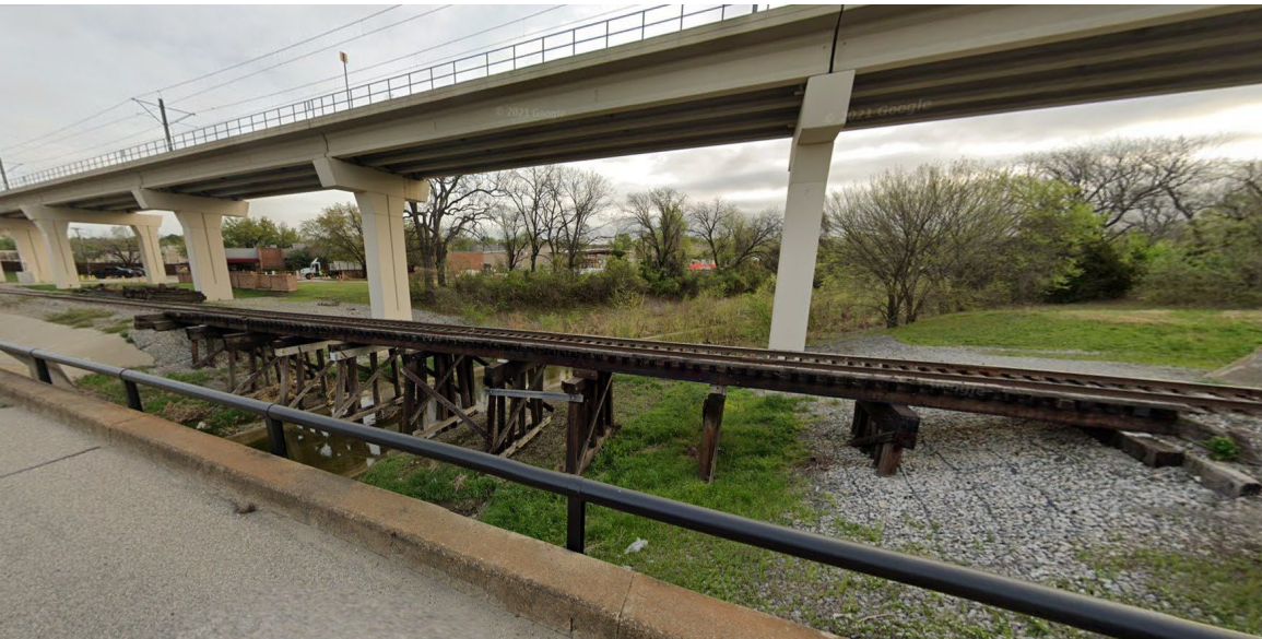
Existing single-track timber trestle over Hutton Branch, beneath the DART Green Line structure.
