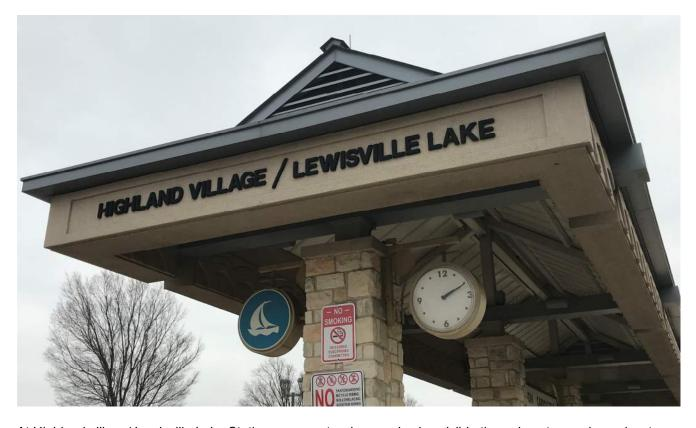
At Highland village/ Lewisville Lake Station some water damage is also visible through water marks and water deposits. Throughout the three canopies, no rust marks or cracks were present at the time this study was conducted.
