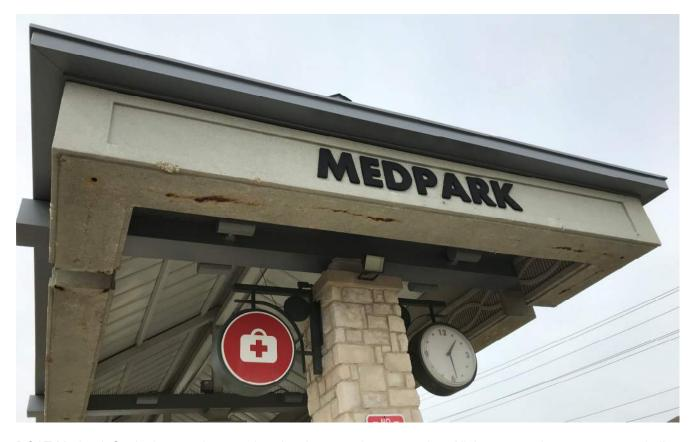
DCAT Medpark Station's canopies are also showing rusted water marks. All three canopies present very similar conditions, rust and water marks along the cracks. At some points finishes are starting to fall off. The extend of the damage to the structural frame is unknown, rust suggests that some steel members might be affected.
