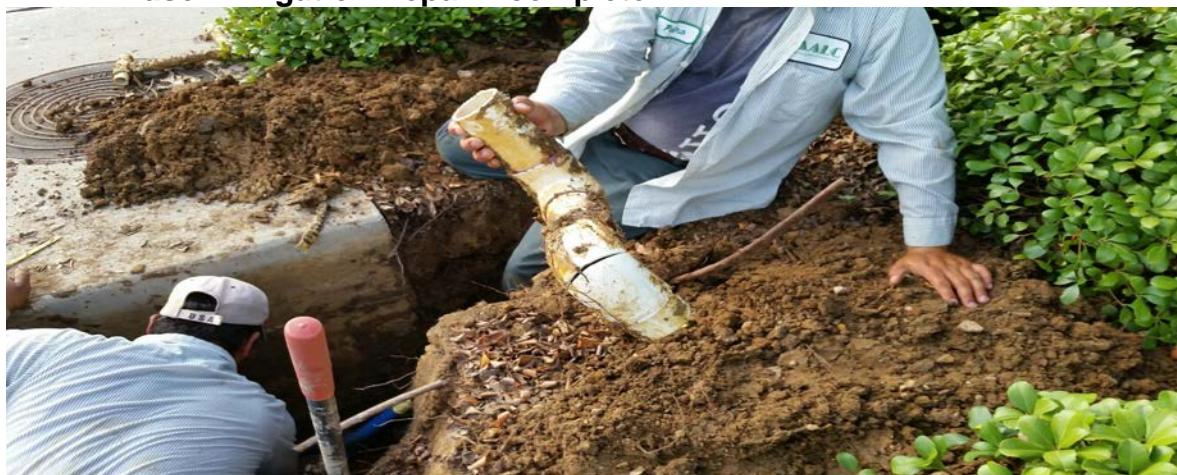
Two inch water line repaired at MedPark station
