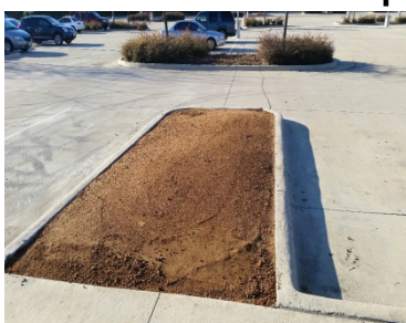
Medpark station: shrubs not suitable for parking areas removed and replaced with deconstructed granite. Alleviates safety/line of site issues.
